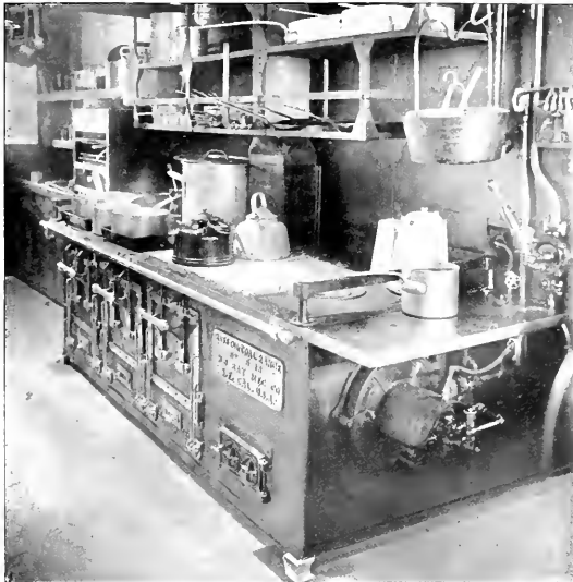
View in the galley of Vanadis showing the Ray portable steel oil burning pumps.
